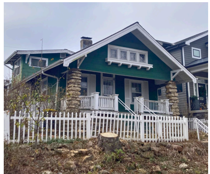
Above: A recently demolished bungalow in the Plaza Westport Neighborhood
