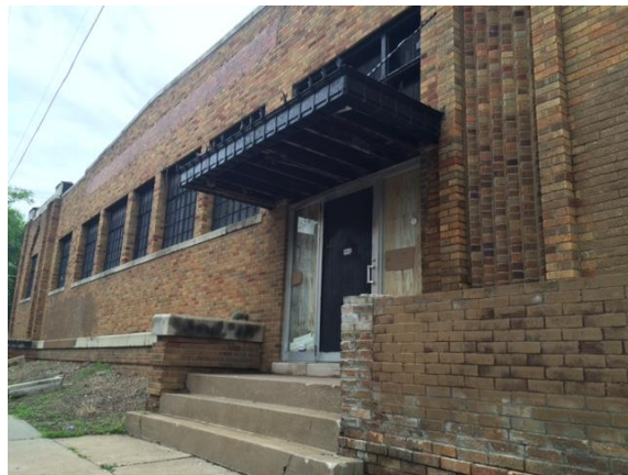
MGM Building, 220-224 W. 18 th Street, Kansas City, MO
