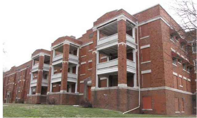
Knickerbocker Apartments at 501-535 Knickerbocker Place
